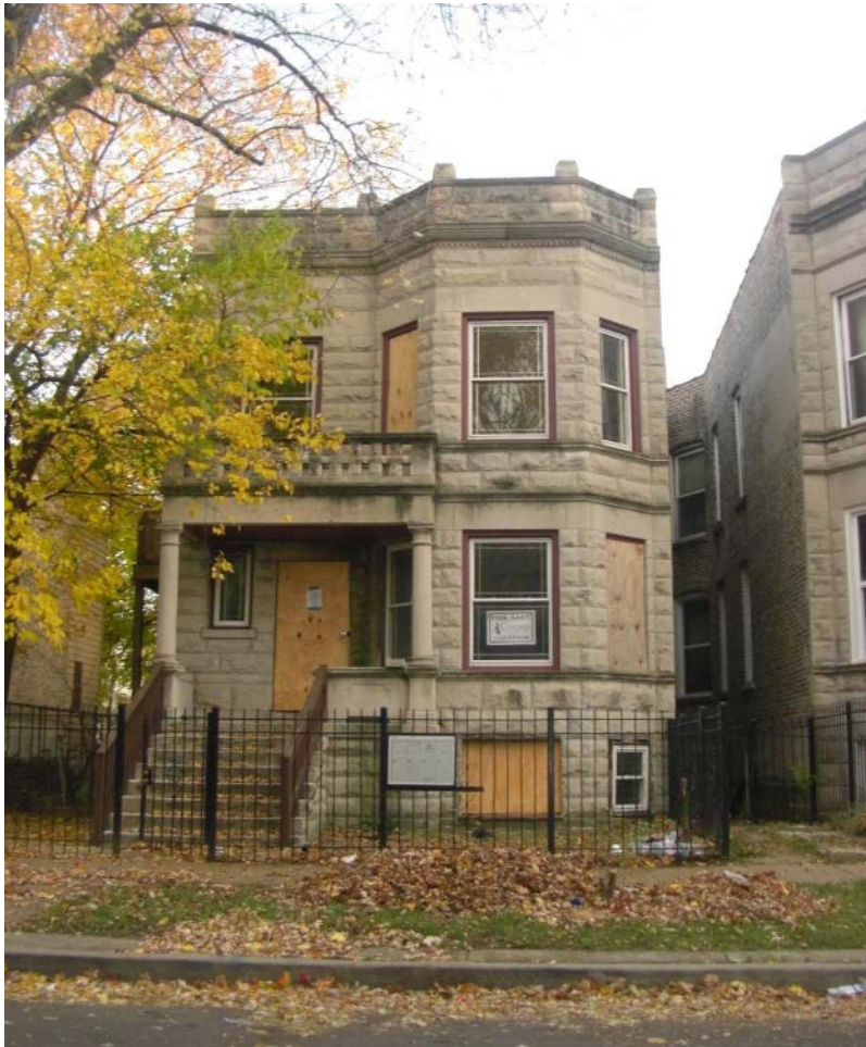
FIGURE 1. Gutted, rehabbed, and abandoned. This classic Chicago grey-stone building dating to the Gilded Age was bought, gutted, and rehabbed like many in West Garfield Park awaiting the arrival of a white market that was slow in coming. Despite its new windows, new gate, new fixtures, and tuckpointing, once it was offered to sell and rent at prices unaffordable to local residents these buildings remain empty and boarded up (photograph by Jesse Mumm).
